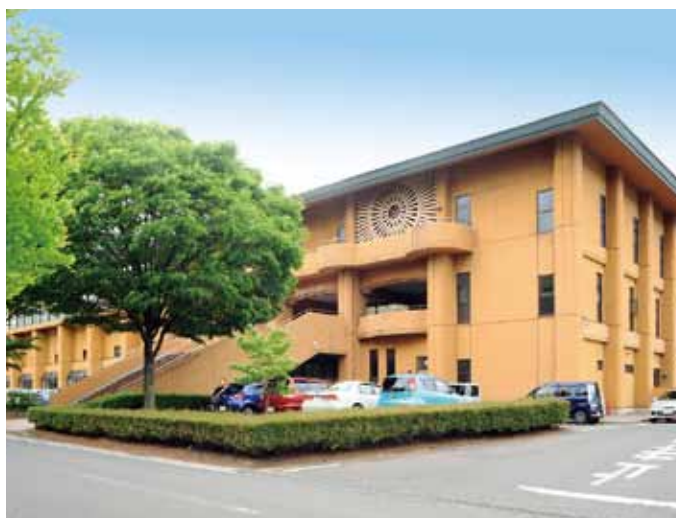
Exterior of Gymnasium
